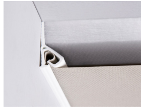
Clipso ceiling installation with PCW profile.
