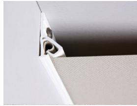
Clipso ceiling installation with PCW profile.
